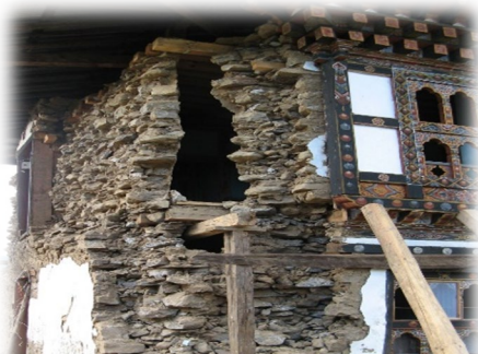
Figure 1. Damage of stone masonry houses during an earthquake
