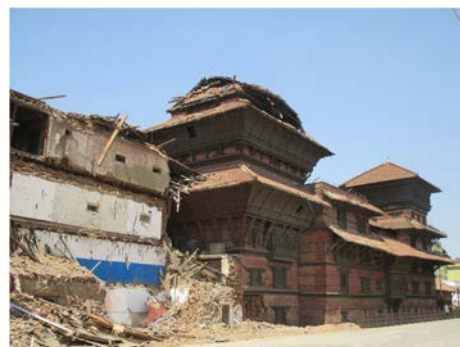
Damage of Kathmandu City (2 June 2015)
