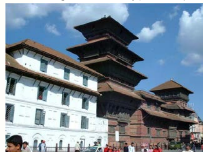
Before 2015 Nepal Earthquake (2006.10)
