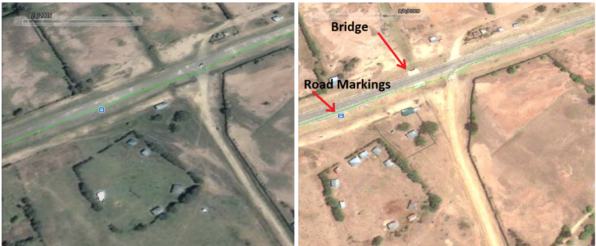
FIGURE 3: VISIBLE IMPROVED ROAD IN KARACHUONYO DISTRICT. Left photo shows the road in 2005 while the right photo shows the road in 2009. Map courtesy of Google ® Maps(0°20'29.66"S34°48'41.26"E)
