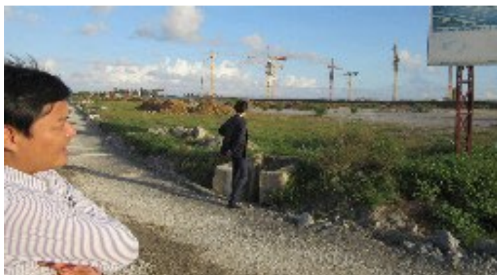
Top-rate hospital construction site in Ha Nam, Vietnam
