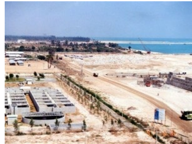
Construction site of Map Ta Phut Industrial Complex in early 1990s (Photo credit: JICA)
